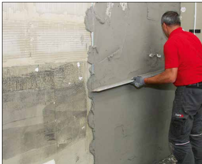
8 Then neatly rule off render by running straightedge over rails from bottom to top.
