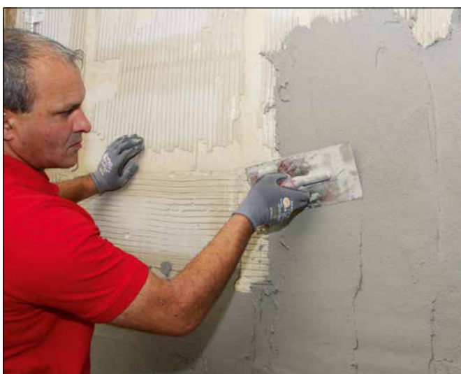
9 Alternatively, RAP 2 434 can be applied using a finishing trowel.
