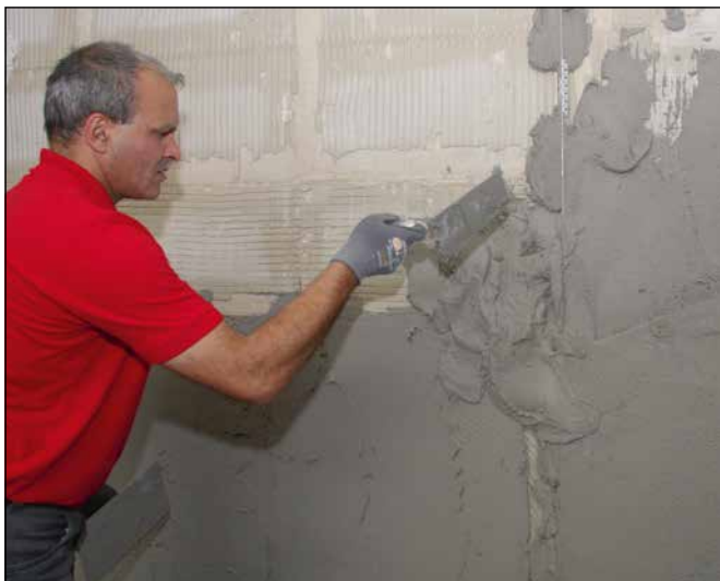
7 Fill area between guide rails by throwing on Sopro RAP 2 434 render.
