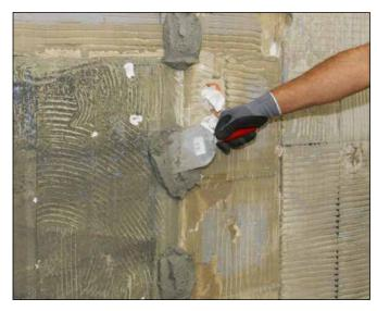
$\boldsymbol{5}$  Fix guide rails for later ruling-off of rendering mortar. Start by applying dabs of render  $\ldots$
