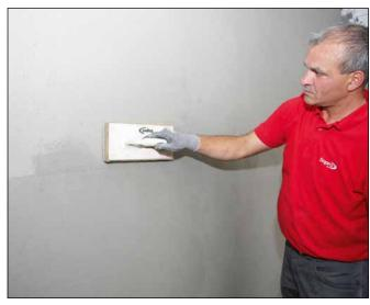
Neatly ruled-off render is ready for tiling after 6 hours. If a tile finish is not required, Sopro RAP 2 434 can be additionally rubbed down with a slightly damp sponge float...
