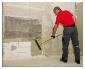
1 Prior to start of works, remove dust and loose particles from substrate.
