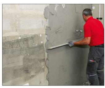
8 Then neatly rule off render by running straightedge over rails from bottom to top.
