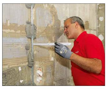
$6\ \dots$  and embed rails at suitable distance from wall, depending on required render thickness, align and allow mortar to set.
