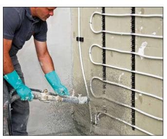
Spray application of Sopro RAP 2 434 is also possible for larger areas, as in pictured example, where render is used to embed (Kermi x-net c21) wall heating system.
