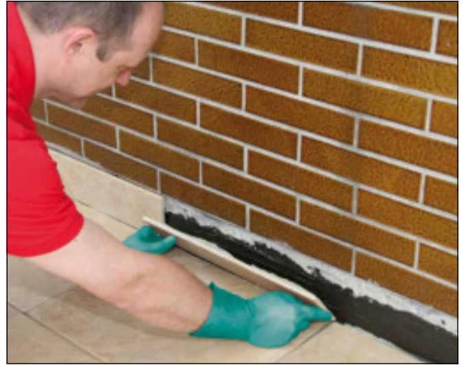
20 ... and place tiles in position.
