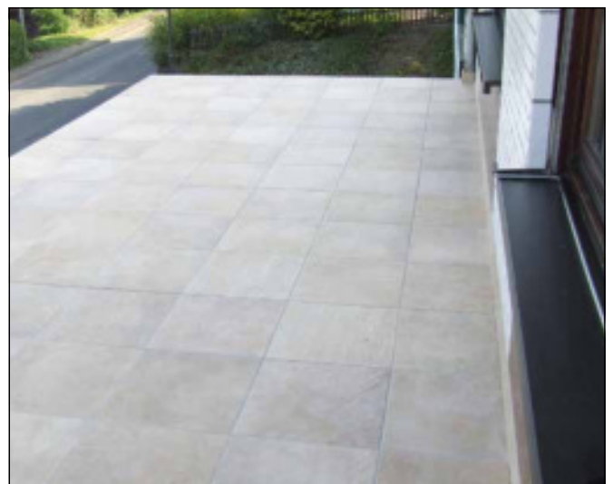
24 Fresh balcony tiling installed using Sopro system components.
