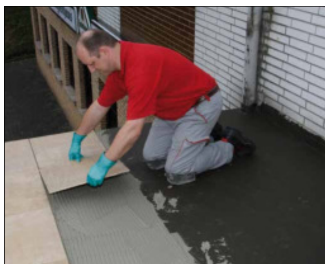
18 Place tiles in freshly placed adhesive bed and align.
