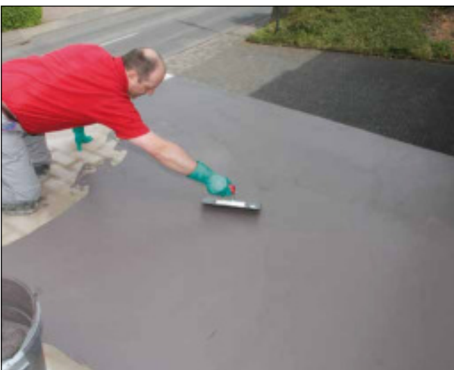
11 Smooth down Sopro TDS 823 with finishing trowel.
