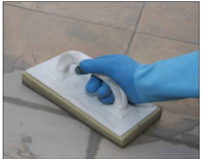
22 Allow adequate drying time for applied Sopro grout, then wash down tiled surface.
