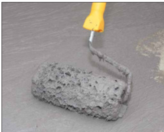
13 Sopro TDS 823 can also be applied using a lambswool roller.
