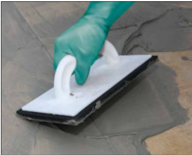
21 After Sopro flexible adhesive has set, finish joints using Sopro tile grout (e.g. Sopro DF 10 flexible designer tile grout or Sopro FL flexible tile grout).
