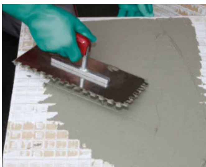
17 Use of buttering/floating method to achieve fullest possible bedding and bonding of covering depends on tile size and nature of rear face.
