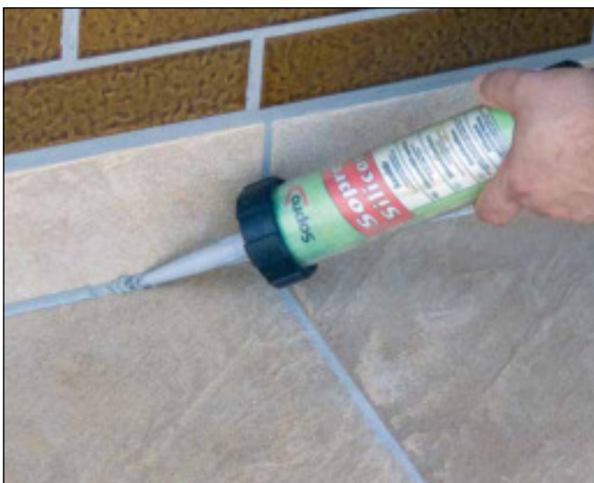
23 Apply Sopro Sanitary Silicone sealant at perimeter and movement joints.
