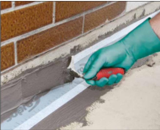
9 Overcoat edges of Sopro DB 438 sealing tape with Sopro TDS 823.
