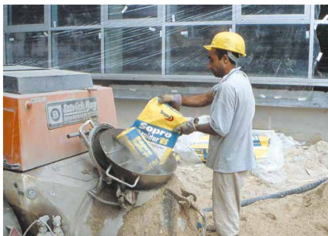
Easy-to-use Sopro Rapidur® B5 binder with straightforward proportioning for on-site preparation.
