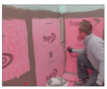
Tape over joints in Sopro AEB 640 membrane with Sopro AEB 148 flexible sealing tape.
