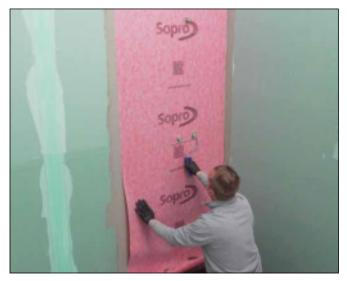
7 Embed accurately cut-to-size Sopro AEB 640 waterproofing and separating membrane in fresh adhesive coat and press down firmly to smooth, working outwards from centre.
