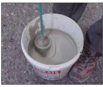
2 Place liquid Component B in container, add full quantity of powder Component A and mix mechanically to lump-free consistency.
