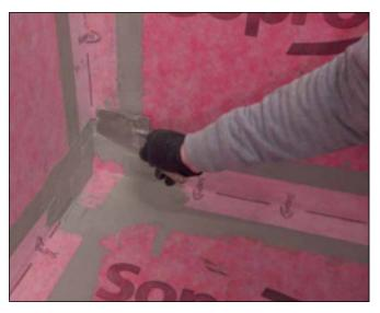
12 Likewise overcoat ends of Sopro AEB 148 tape sheet with Sopro FDK 415.
