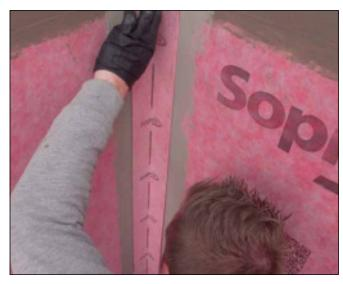
11 Embed accurately cut-to-size Sopro AEB 148 tape in fresh adhesive coat and press down firmly.
