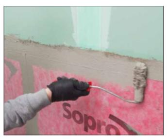
Overcoat Sopro AEB 640 sheet terminations with Sopro FDK 415.
