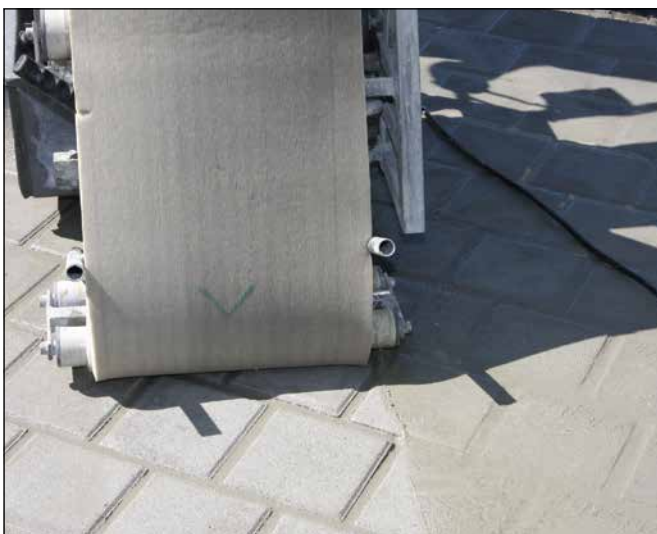
5 Washing down of pavement with cleaning machine ...
