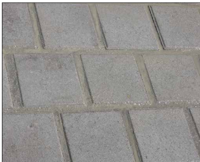
8 Grouted concrete segmental pavement.
