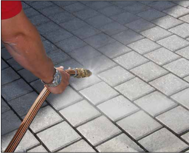
1 Pre-wetting of cleaned pavement to be grouted.
