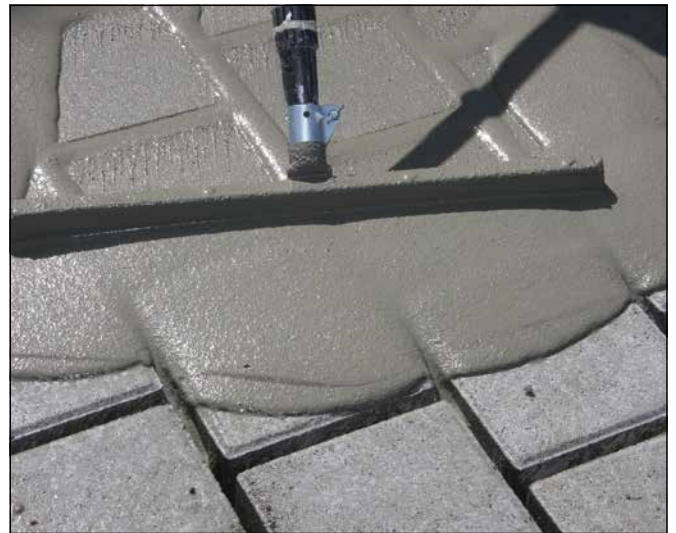
4 Filling of joints with Sopro BSF 611.
