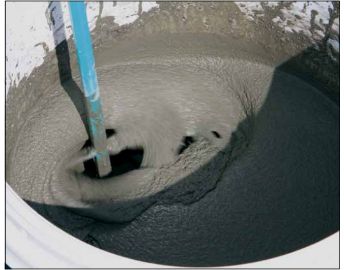
2 Preparation of Sopro BSF 611.
