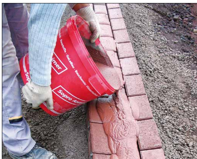
2 Application of suitably tinted Sopro BSF 611.
