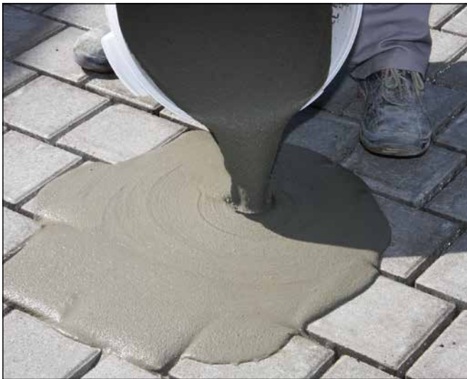
3 Pouring of Sopro BSF 611 onto pavement.
