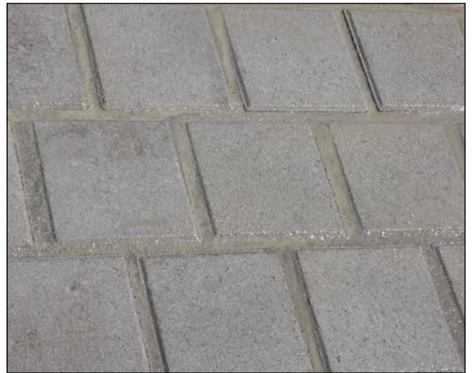
8 Grouted concrete segmental pavement.
