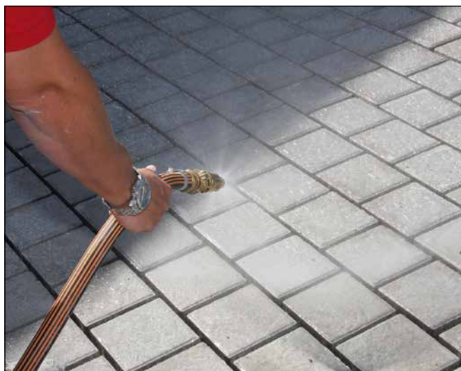
1 Pre-wetting of cleaned pavement to be grouted.
