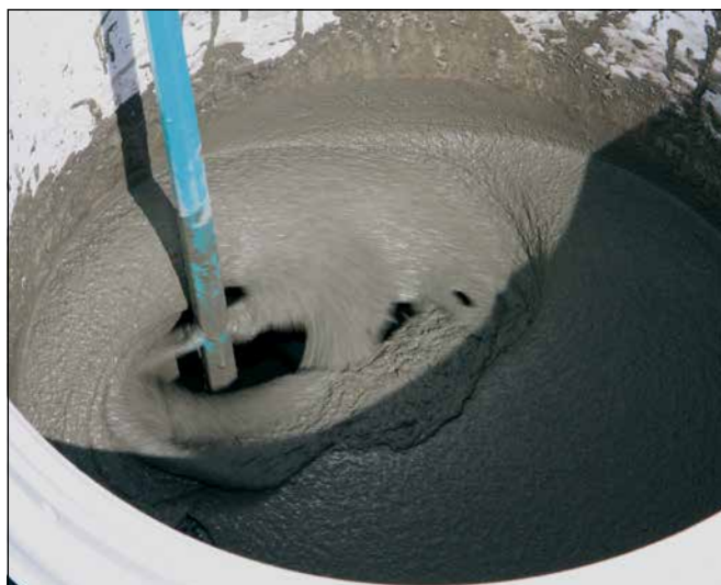
2 Preparation of Sopro BSF611.
