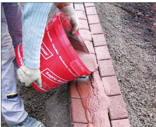
2 Application of suitably tinted Sopro BSF 611.
