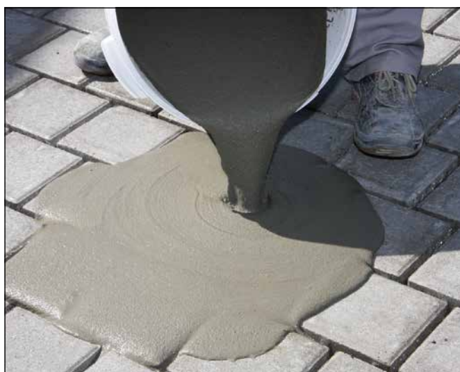
3 Pouring of Sopro BSF611 onto pavement.
