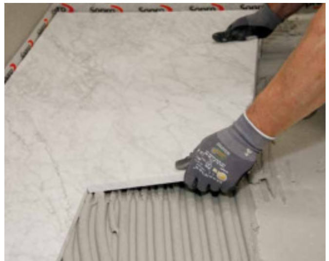
2 Laying of natural stone unit. Due to its light colour, Sopro FKM 600 is also suitable for laying translucent materials.
