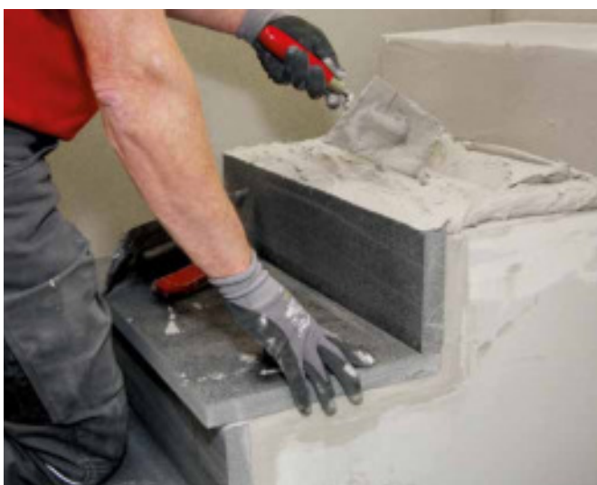
1 Sopro FKM 600 can also be applied in greater coat thicknesses of up to 20 mm.
