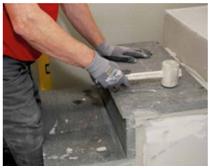
2 Installation of step. Rapid-set properties of adhesive allow early loading.
