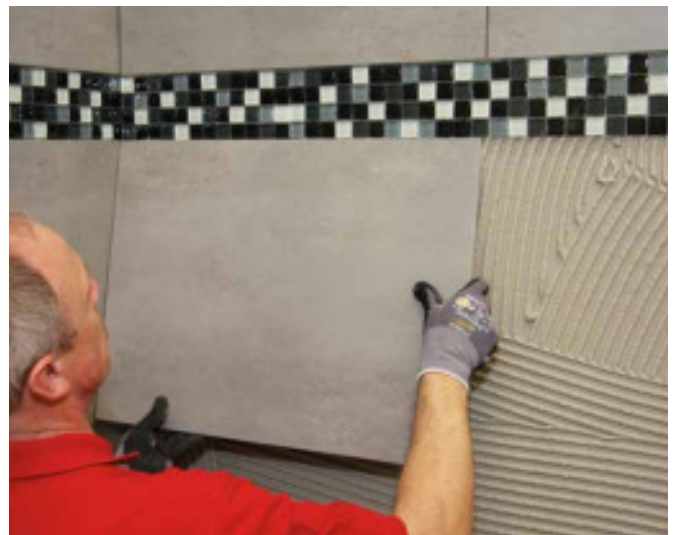
4 Easy wall installation of large-format fully vitrified stoneware units due to high sag resistance.
