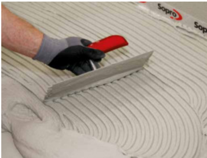
1 Application of contact layer and combed bed in floating-bed consistency.
