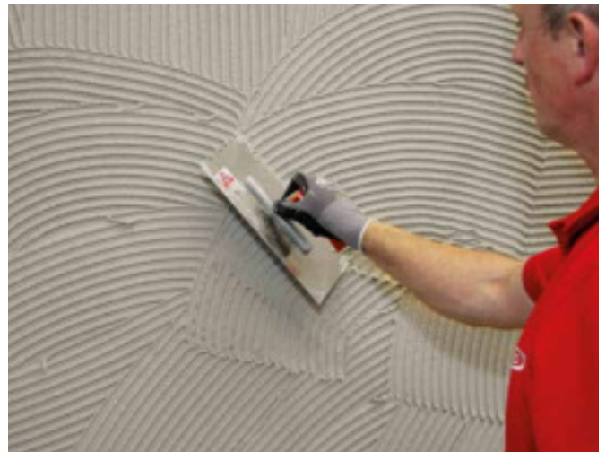
2 Application of contact layer and combed bed in thin-bed consistency.
