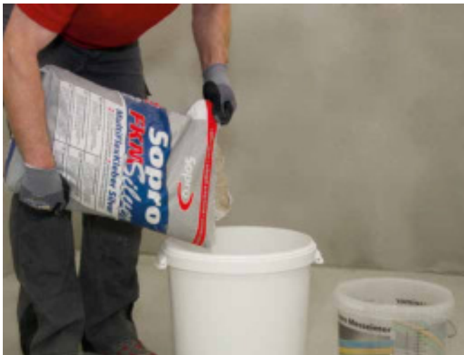
1 Mixing of Sopro FKM 600 to required consistency for thin-bed, floating-bed or medium-bed laying or for surface filling.
