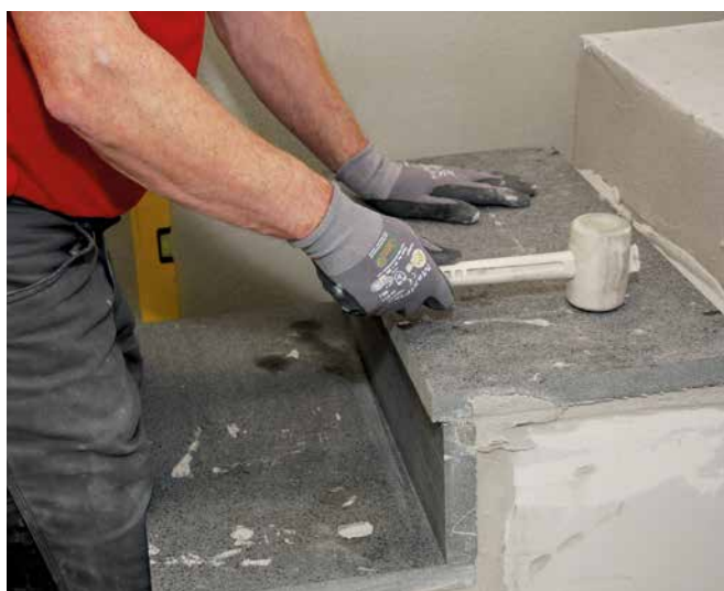
2 Installation of step. Rapid-set properties of adhesive allow early loading.
