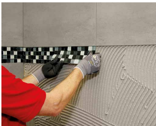
3 Laying of glass mosaic in prepared adhesive bed.
