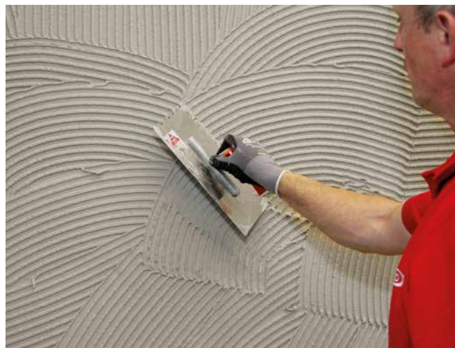
2 Application of contact layer and combed bed in thin-bed consistency.
