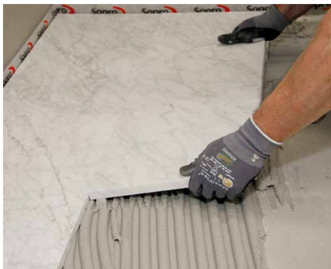
2 Laying of natural stone unit. Due to its light colour, Sopro FKM 600 is also suitable for laying translucent materials.
