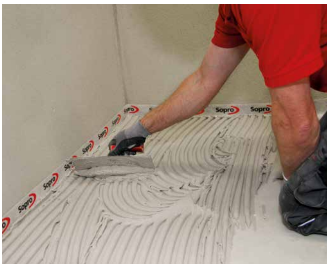
1 Application of Sopro FKM 600 in medium-bed consistency for medium-bed laying.
