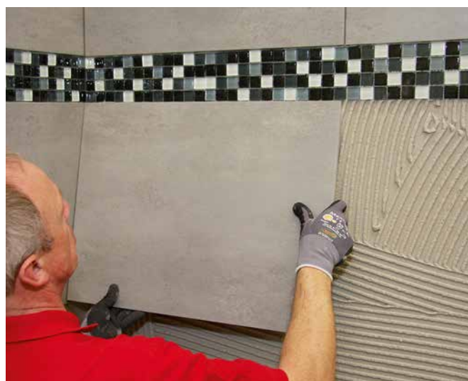
4 Easy wall installation of large-format fully vitrified stoneware units due to high sag resistance.
