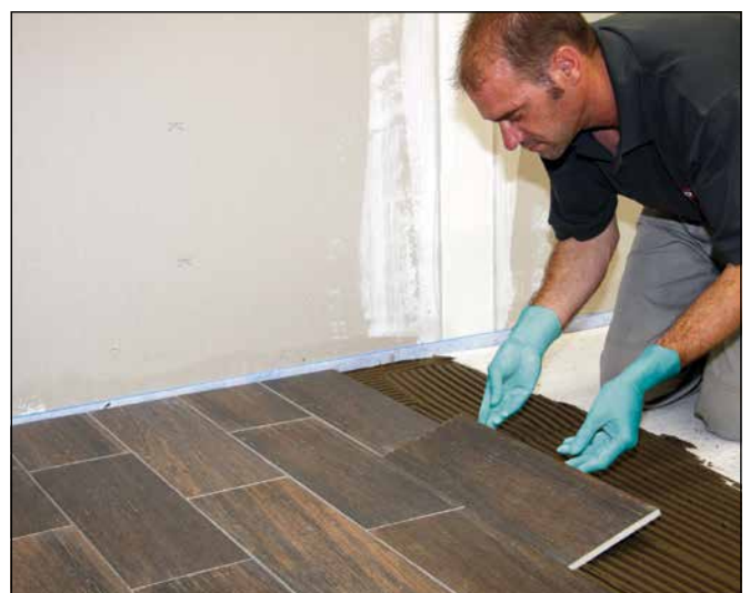
12 Apply Sopro flexible adhesive (e.g. Sopro's No.1) and place tiles.
