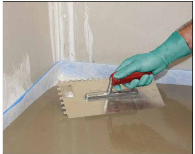
8 Sopro FAS 551 may be spread uniformly using squeegee or finishing trowel.
