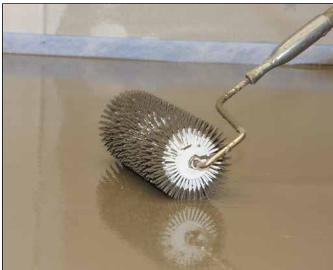
9 A spiked roller may be used to release entrapped air from applied filler compound.
