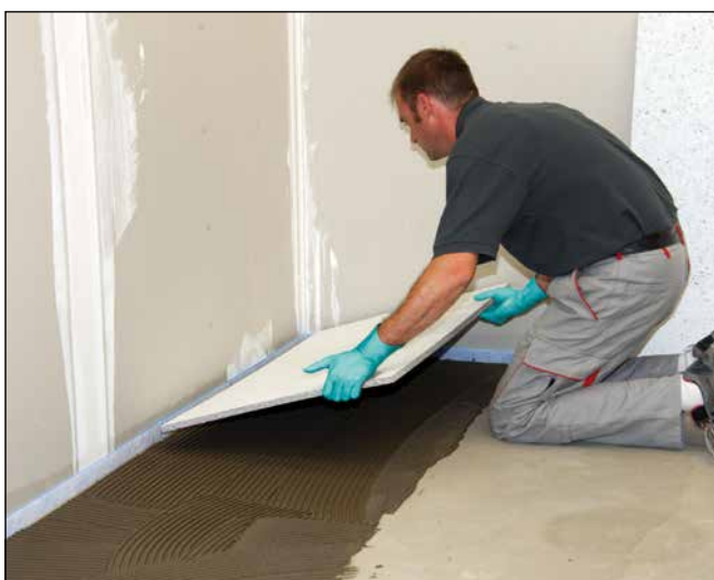
11 To accommodate movement in substrate, subsequent incorporation of Sopro FDP 558 tile insulation board using Sopro flexible adhesive (e.g. Sopro's No.1) is strongly recommended.
