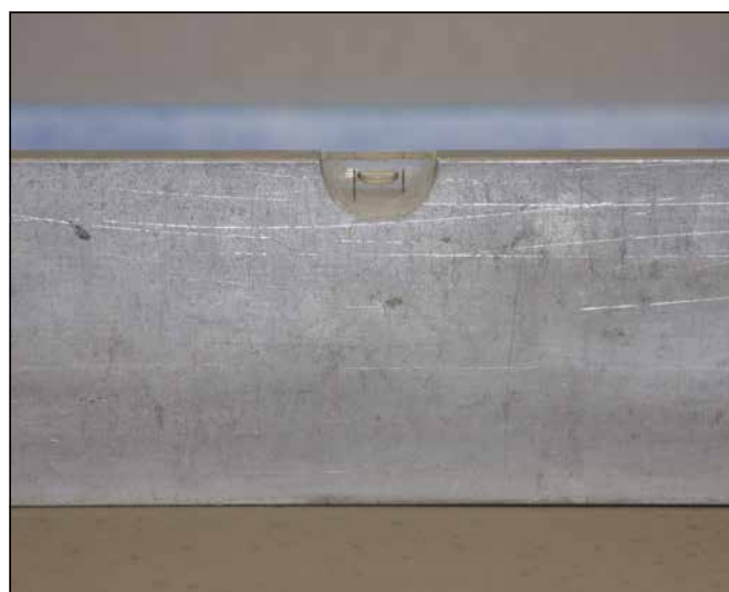
10 Once set, Sopro FAS 551 provides level surface ready to receive floor covering.
