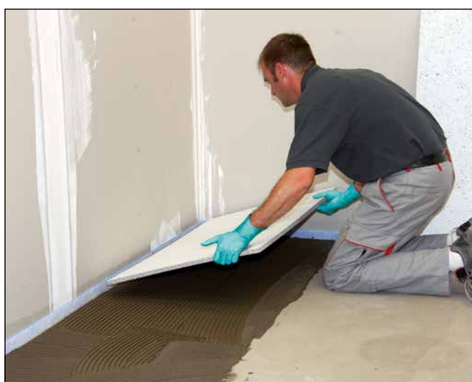
11 To accommodate movement in substrate, subsequent incorporation of Sopro FDP 558 tile insulation board using Sopro flexible adhesive (e.g. Sopro's No.1 400) is strongly recommended.
