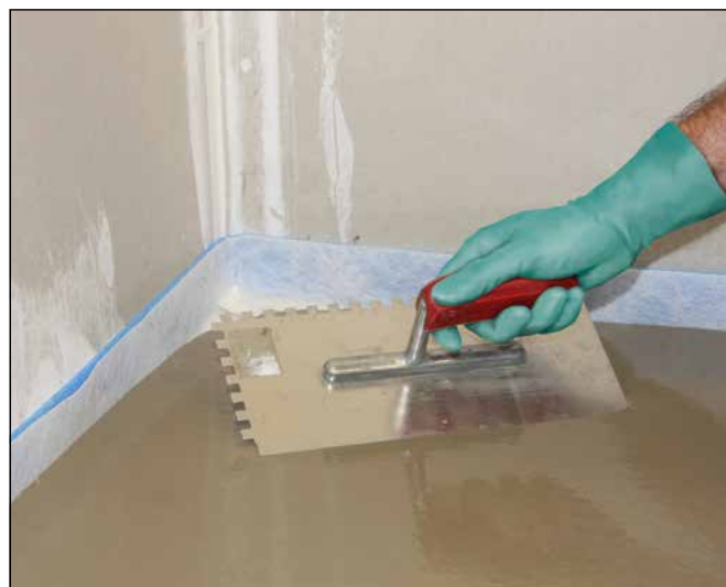
8 Sopro FAS 551 may be spread uniformly using squeegee or finishing trowel.
