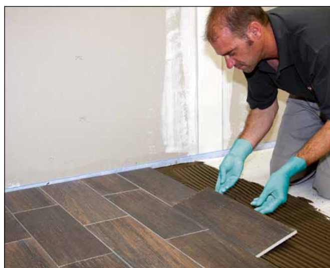
12 Apply Sopro flexible adhesive (e.g. Sopro's No.1 400) and place tiles.
