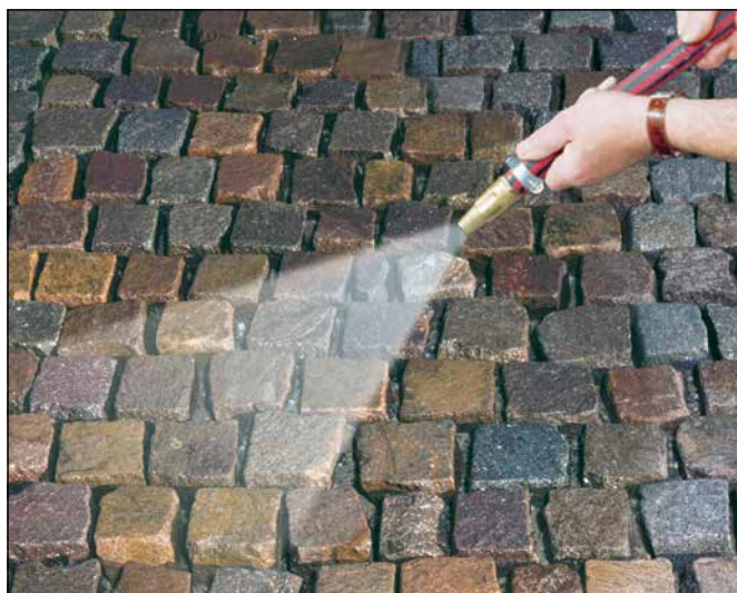
1 Pre-wet cleaned pavement to be grouted.
