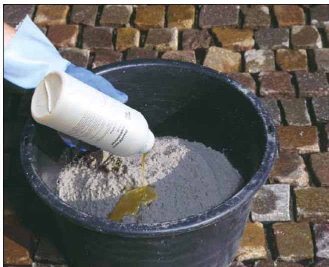
2 Add curing agent and stir Sopro EPF.
