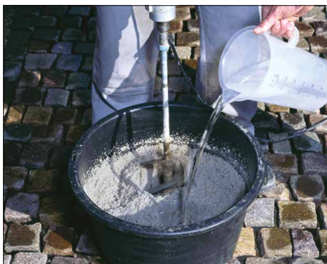
3 After preparation of Sopro EPF, add approx. 2 ltr water and restir.
