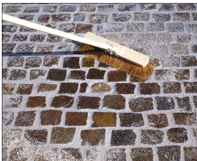
6 Clean grouted pavement.
