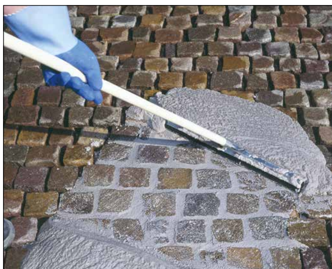
5 Fill joints with Sopro EPF.
