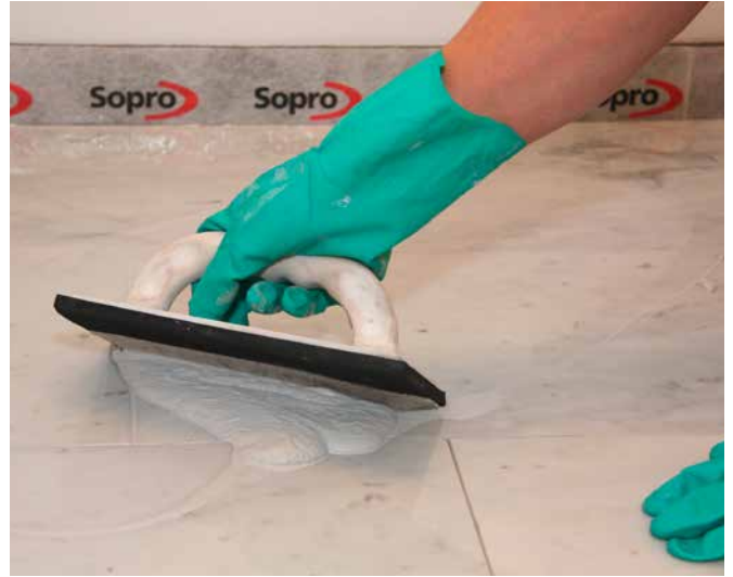
8 Grouting of discoloration-sensitive natural stone with Sopro DF 10®.
