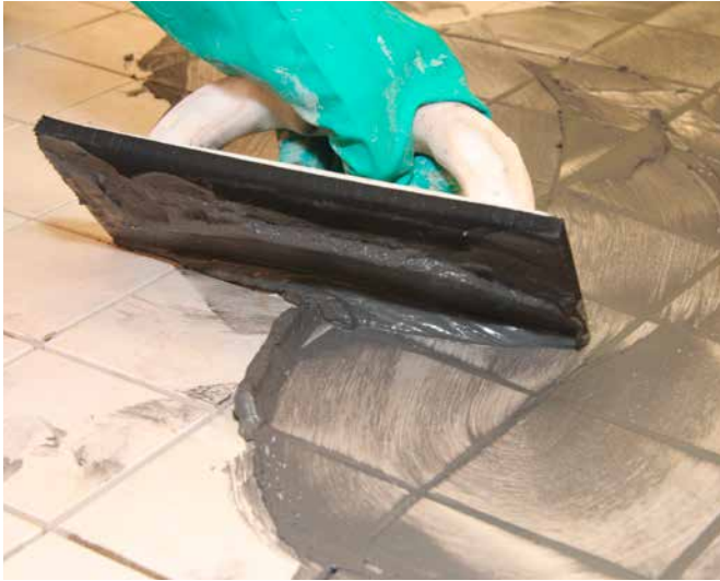
7 Grouting of fully vitrified stoneware tiles with Sopro DF 10®.
