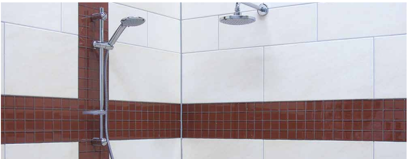
11 Brilliantly coloured joint surfaces in bathroom.
