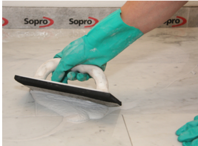
8 Grouting of discoloration-sensitive natural stone with Sopro DF 10®.
