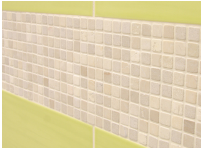
10 Earthenware and natural stone mosaic surfaces grouted with Sopro DF 10®.
