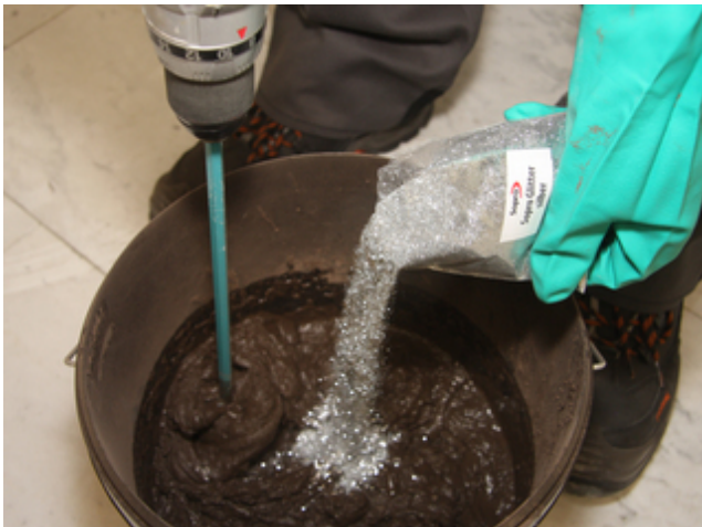
3 If required, up to 2 bags of Sopro glitter may be added to grout during mixing. If glitter is added, increase proportion of water.
