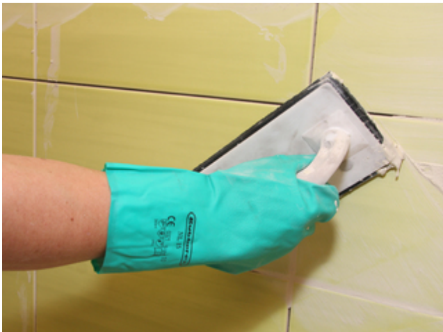
9 Grouting of earthenware tiles with Sopro DF 10®.
