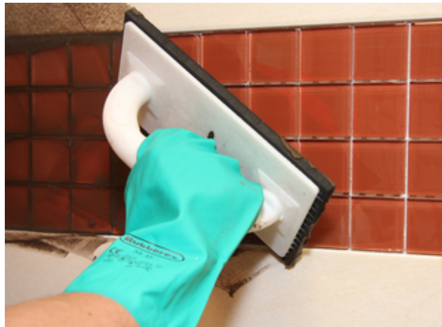
4 Grouting of glass mosaic using Sopro DF 10 ® with Sopro silver glitter.
