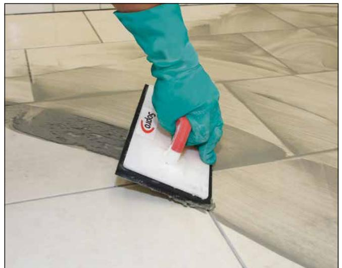
**16** Finish joints with Sopro tile grout (e.g. Sopro DF 10 flexible designer tile grout or Sopro Brilliant® water-repellent tile grout).
