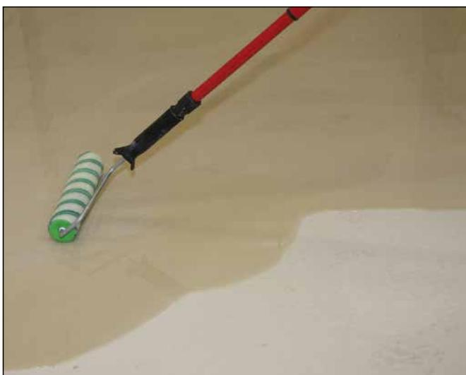
**11** ... spread reaction resin primer using Sopro short-pile roller to form thin film, taking care to avoid ponding ...
