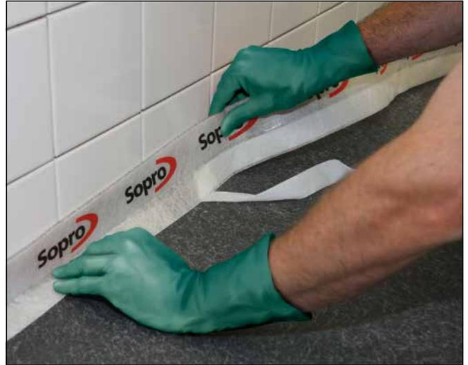
2 When Sopro HPS 673 has dried (after 1–2 hours), fix self-adhesive Sopro RDS 960 perimeter insulation strip.
