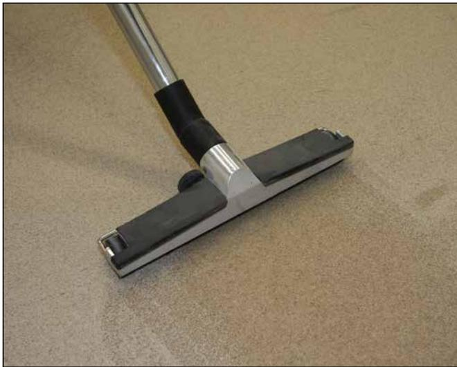
**13** After Sopro EPG 522 or Sopro MGR 637 has fully dried (after approx. 24 hours or 30–40 minutes respectively), use industrial vacuum cleaner or broom to remove surplus silica sand.
