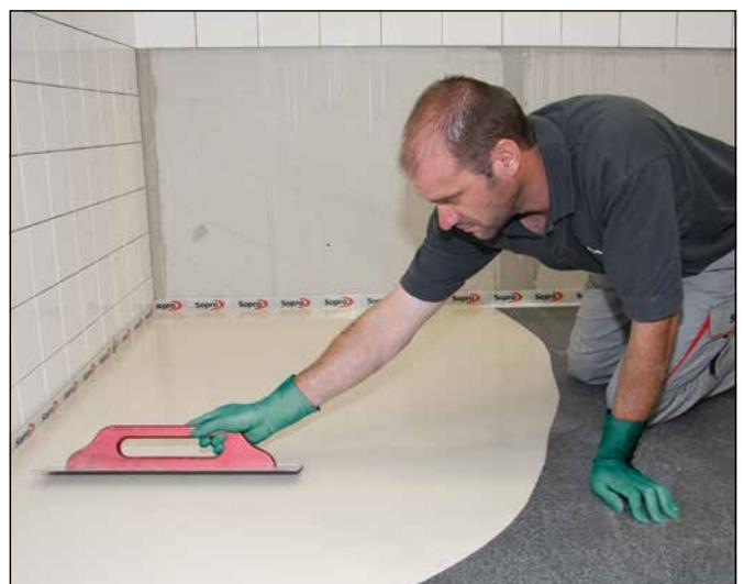
6 Spread Sopro AFS 561 uniformly to required coat thickness using squeegee or finishing trowel.
