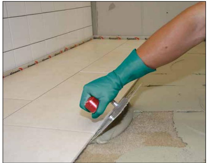
**14** Apply Sopro flexible tile adhesive (e.g. Sopro FKM 444 XL, Sopro VF XL 413) to dried primer coat.
