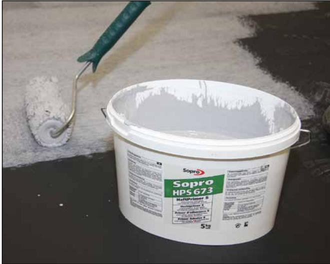
1 Roll Sopro HPS 673 bonding primer onto unblinded mastic asphalt screed. Sopro GD 749 primer is recommended for pretreatment of absorbent substrates (e.g. anhydrite screeds).
