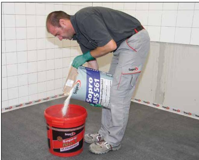
3 Fill mixing bucket with specified quantity of water and add Sopro AFS 561.
