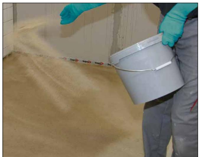
**12** ... and blind with 0.4–0.8 mm Sopro QS 511 coarse silica sand.
