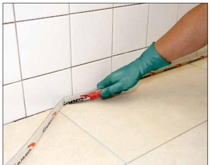
**18** Cut off top of Sopro RDS 960 perimeter insulation strip with utility knife.
