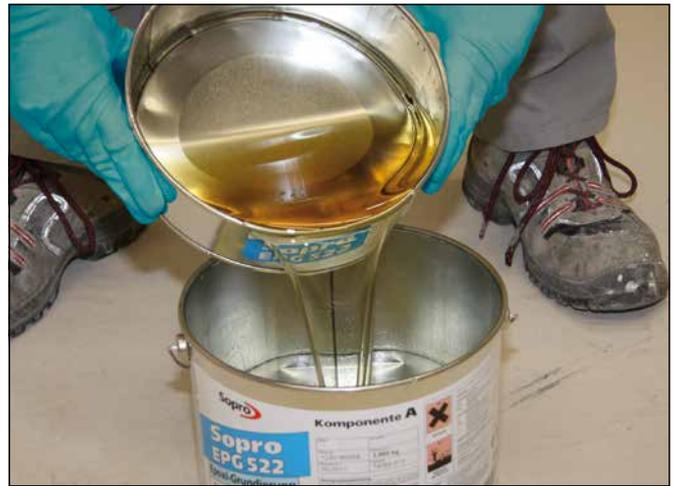
**8** Pretreat surface with Sopro EPG 522 epoxy primer or (one-component) Sopro MGR 637 multi-purpose primer to prevent moisture migration back into anhydrite screed construction. Add all Sopro EPG 522 Component B to container with Component A and mix to homogeneous consistency.
