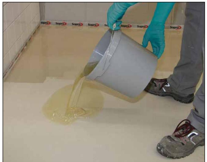
**10** When substrate coated with Sopro AFS 561 is walkable and has been CM tested for residual moisture, pour on Sopro EPG 522 or Sopro MGR 637 ...
