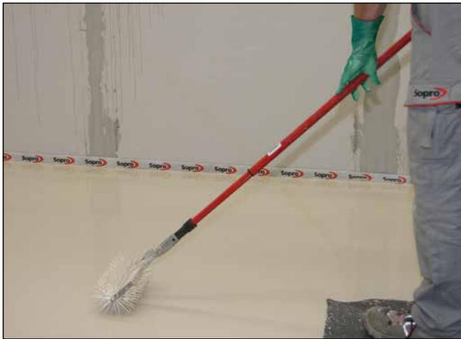
**7** A spiked roller may be used to release entrapped air from freshly applied levelling compound. Before proceeding with installation, allow Sopro AFS 561 to dry for min. 24–36 hours and perform CM measurement to determine residual moisture.
